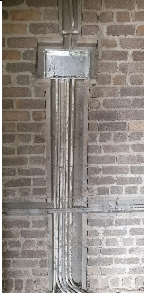
Photograph 5: Installation of DB board
